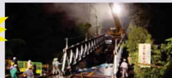
Construction of temporary bridge
