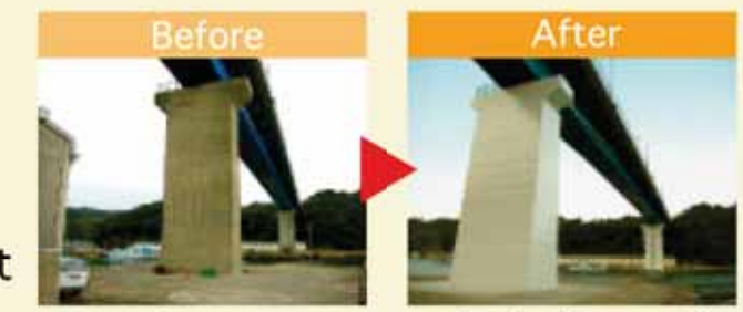
Pier enforcement, Kannoura-bridge (Route 55)
