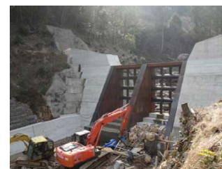
○生名谷川砂防堰堤
