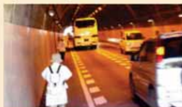
Awa Tunnel without sidewalk (Route 56)
