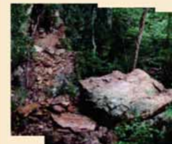
Broken rock by cracking (Hill along Route 32)
