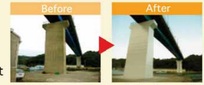
Pier enforcement, Kannoura-bridge (Route 55)
