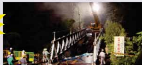
Construction of temporary bridge
