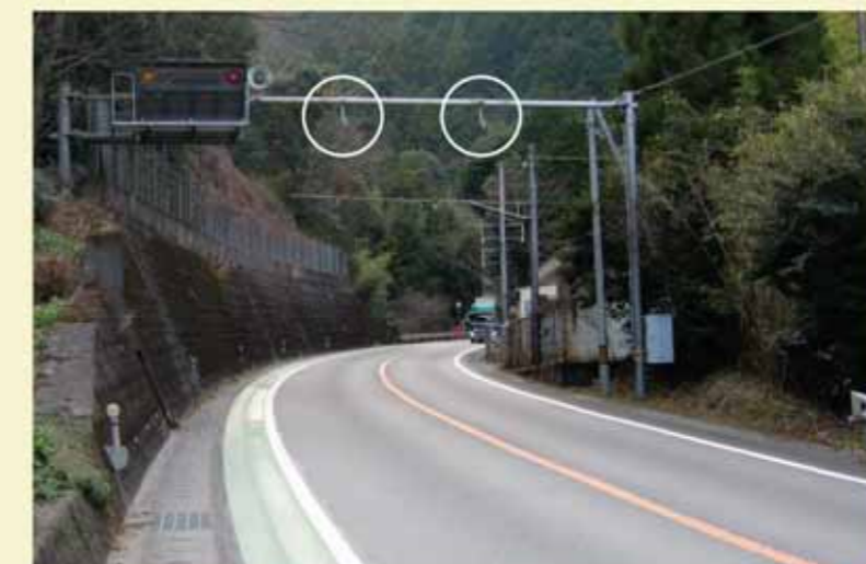
Continual observation by traffic counter (Yakezaka, Route 56)
