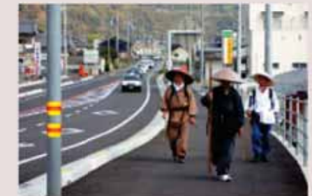
Ioki road for pedestrian and bicycle users
