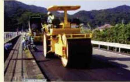
Repair of road pavement
