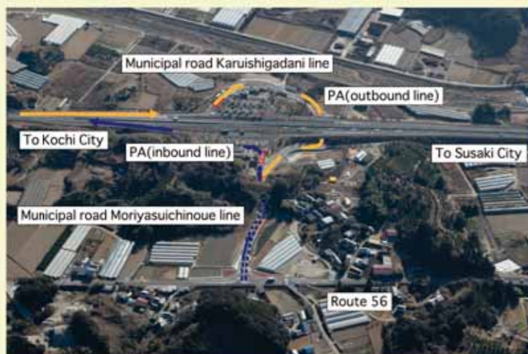
Tosa parking area Smart-IC (Kochi expressway)
