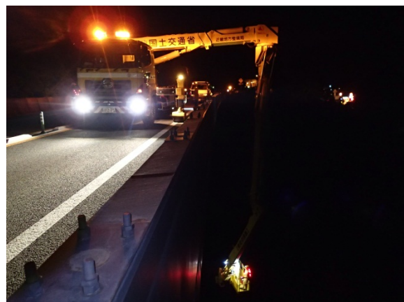
⑤橋梁点検
