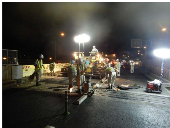
②路面補修
