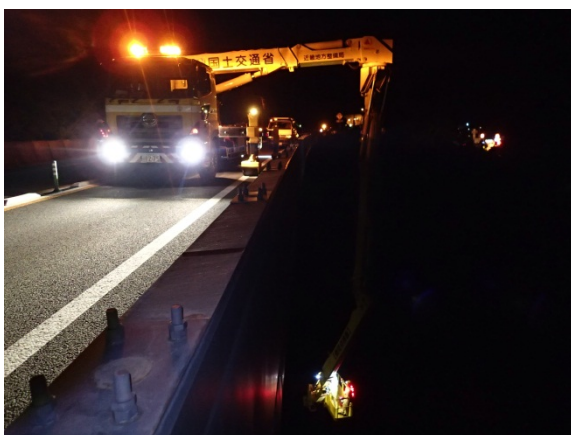
⑤橋梁点検
