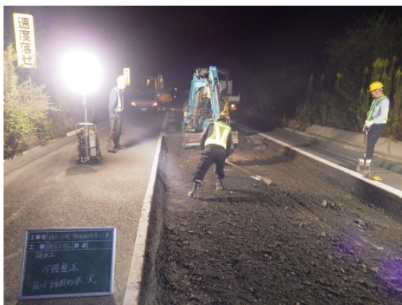
②路面補修
