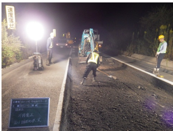
②路面補修
