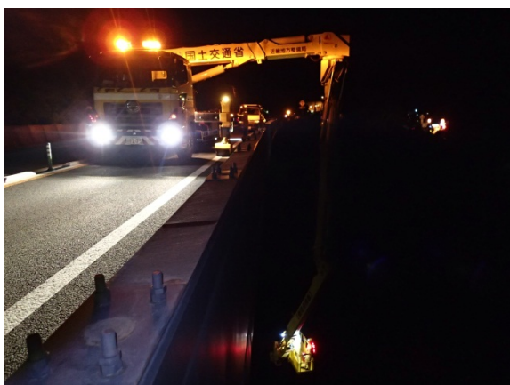
⑤橋梁点検
