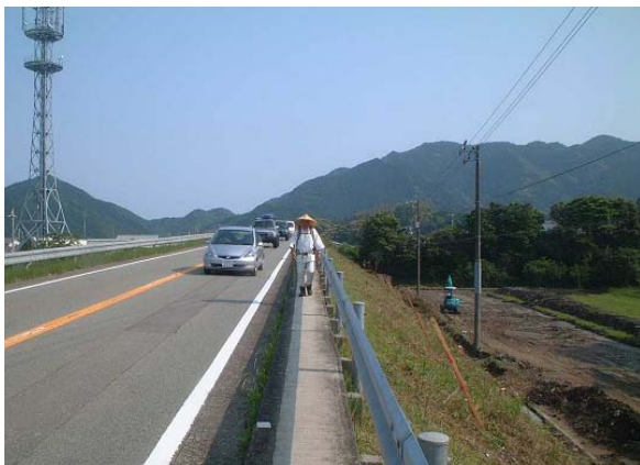
歩道拡幅前 W=0.75m (整備前)
